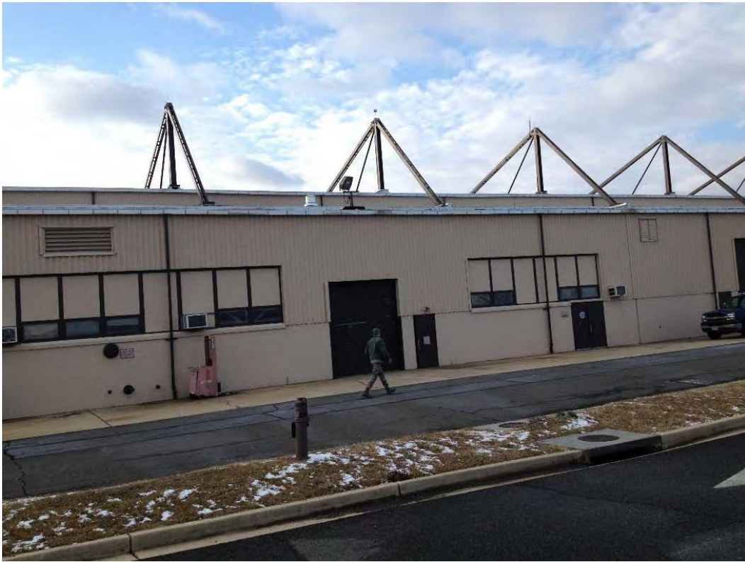
Photo 2: View of back of Hangar 14 facing west.
