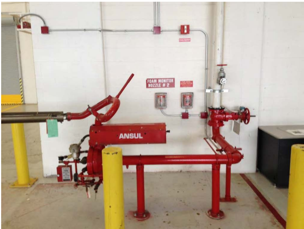
Photo 2: View of Hangar 10 floor cannon.
