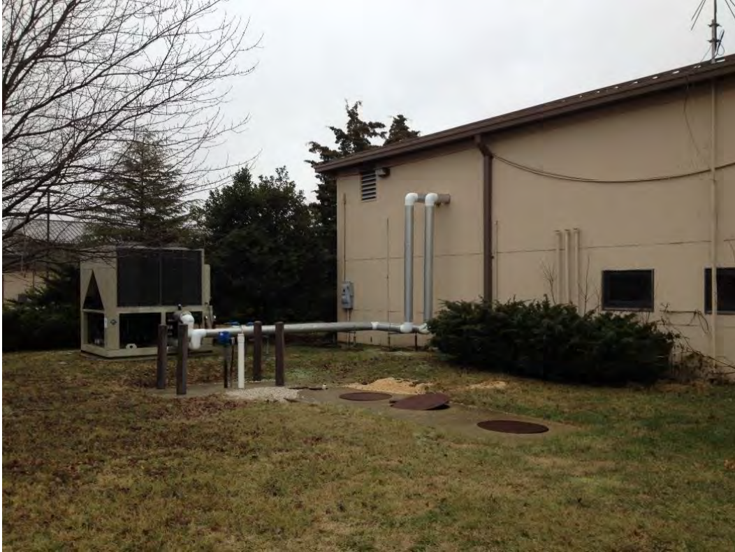
Photo 1: View of northeast corner of Hangar 8. Location of containment system.
