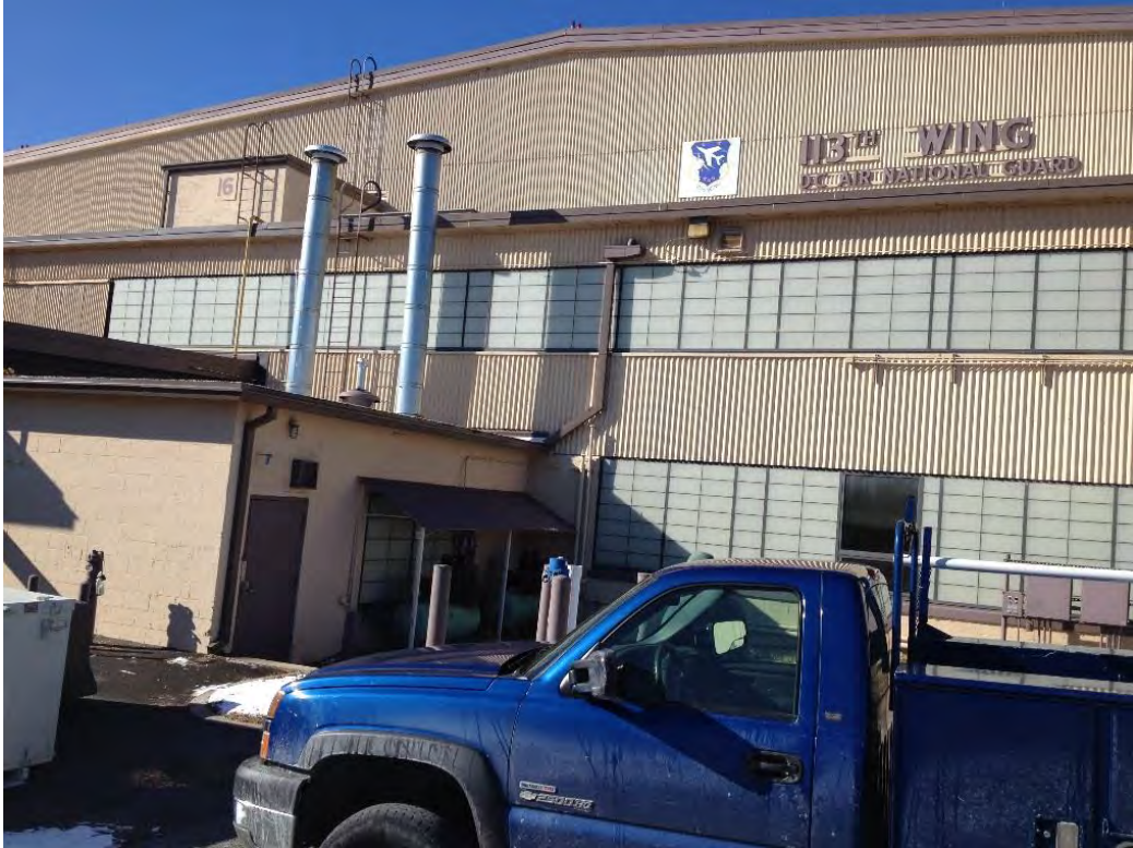
Photo 1: View of Hangar 16 facing west with isolation containment captured in photo.
