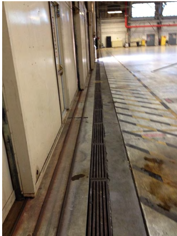
Photo 2: View of trench drain in Hangar 5.
