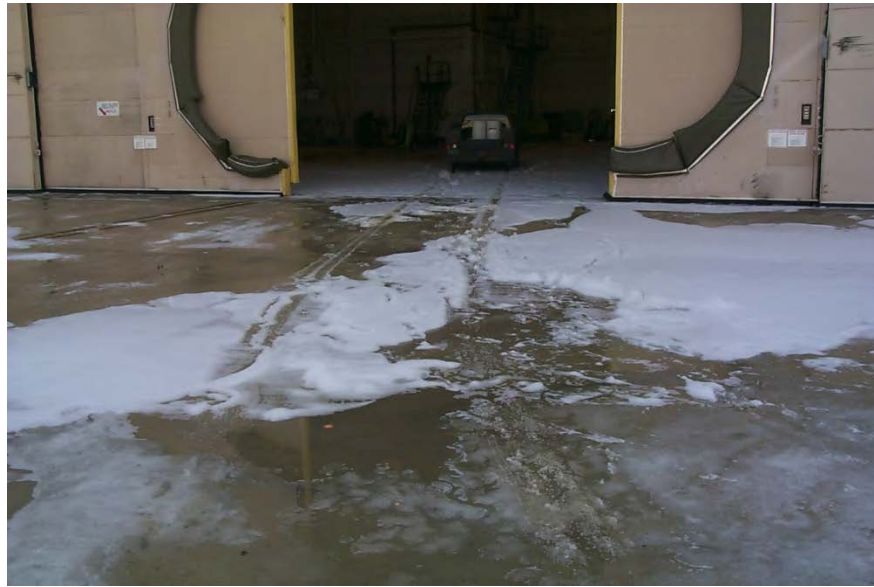
JBA provided photo of circa 2000-2001 timeframe AFFF release at building 3629 on Apron
