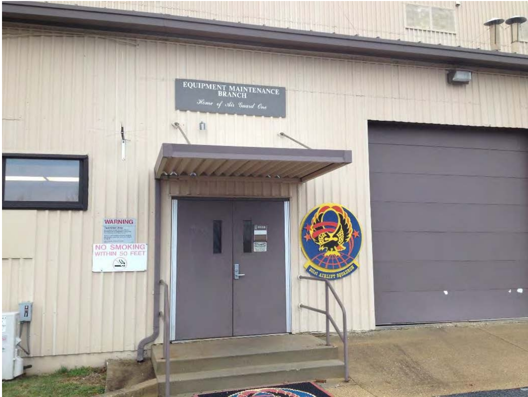
Photo 1: View of Hangar 9 exterior.
