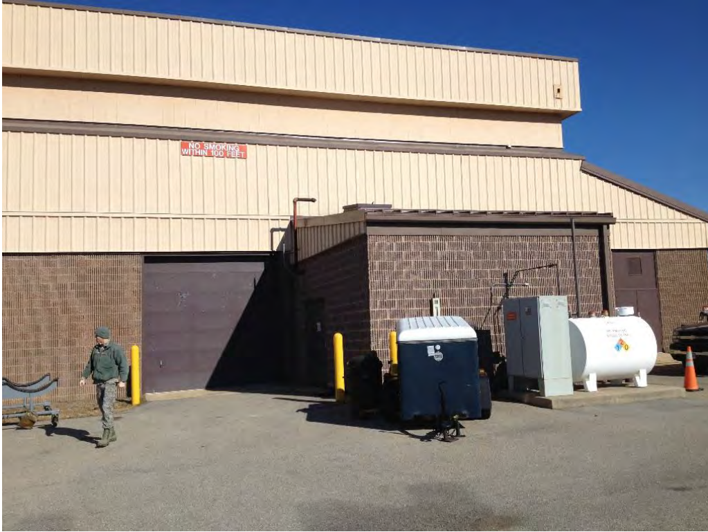
Photo 1: View of BLDG 3302 exterior photo of MEC room facing north.
