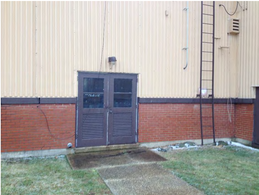
Photo 2: View of Hangar 4 MEC room entrance on east side of Hangar.
