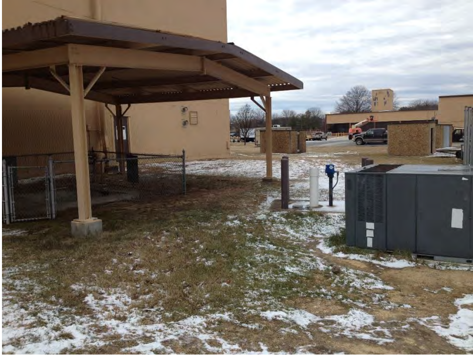
Photo 1: View of north side West Fuel Cell facing west.
