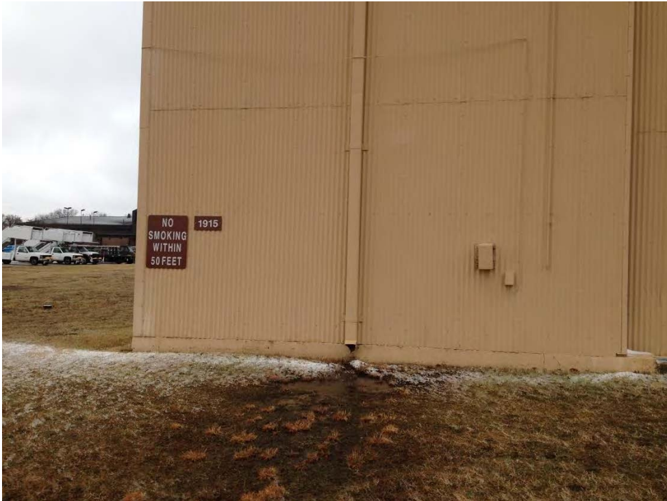
Photo 2: View of West Fuel Cell, front of BLDG facing west.
