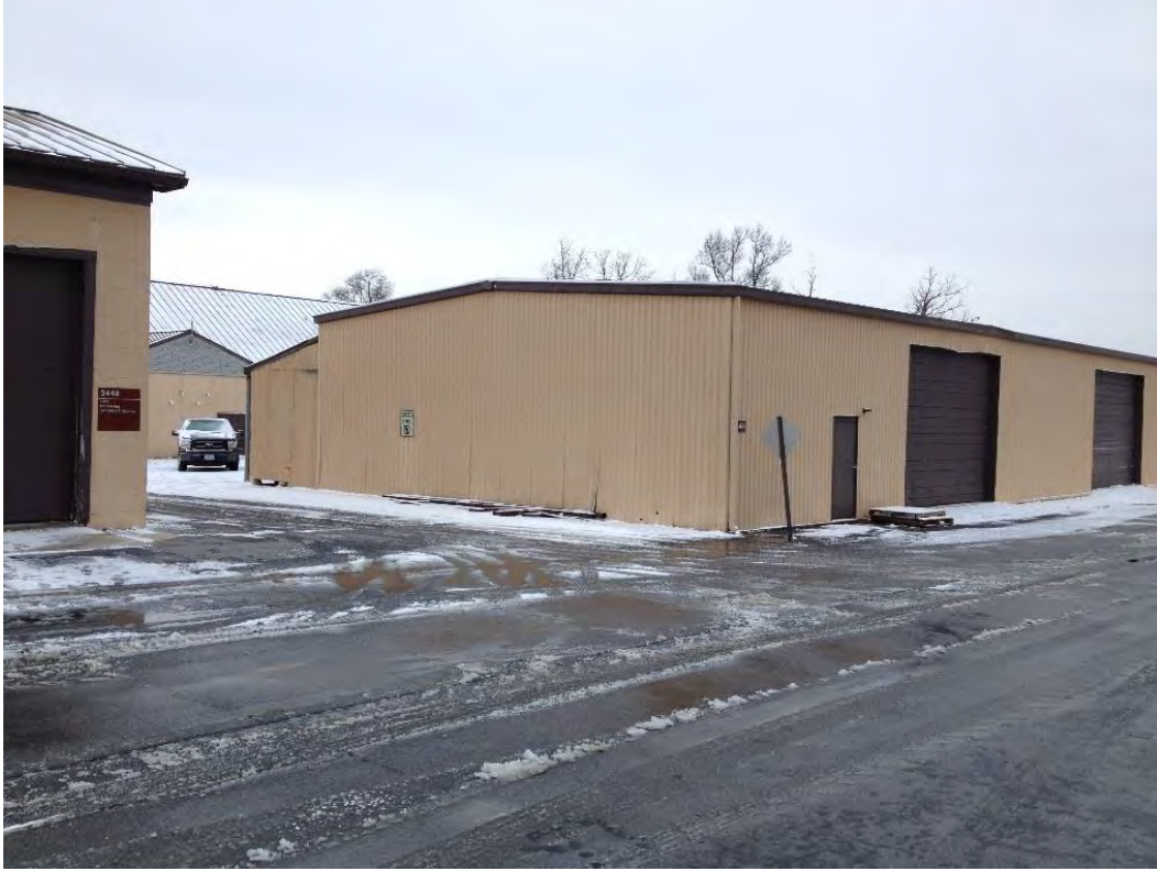
Photo 1: View of BLDG 3444 facing northwest.
